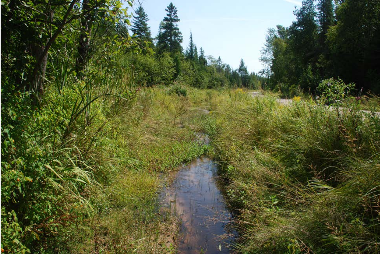
Plate 13. Epoufette ditch along Epoufette Bay Road.
